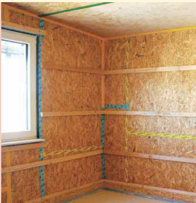
Airtight connections between wood composite boards
