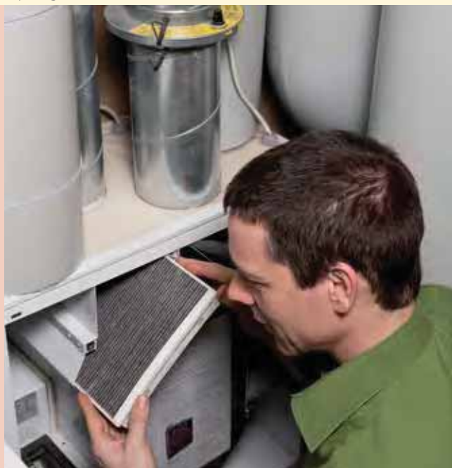
Replacing the filter of a ventilation unit.
